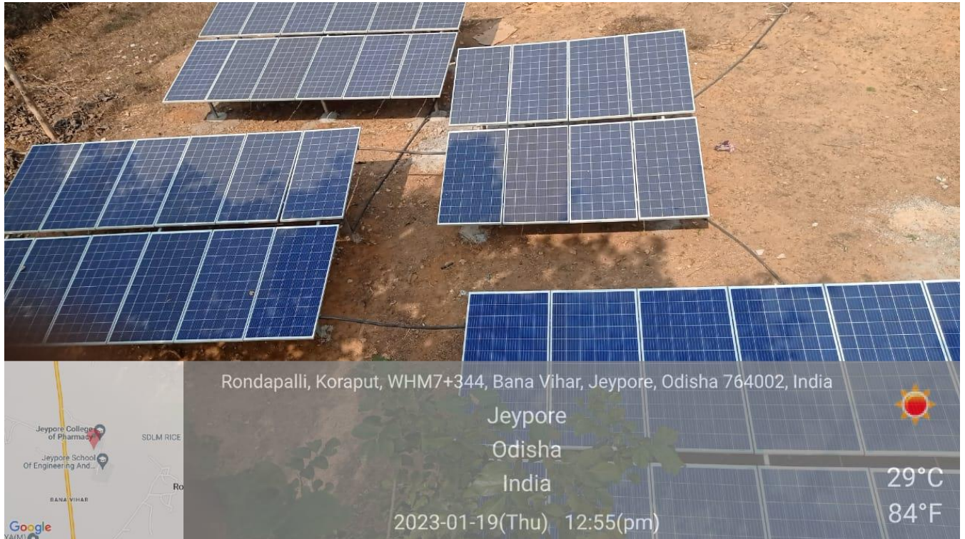
Fig-1 Solar Unit(15KW) installation at Jeypore college of Pharmacy.
