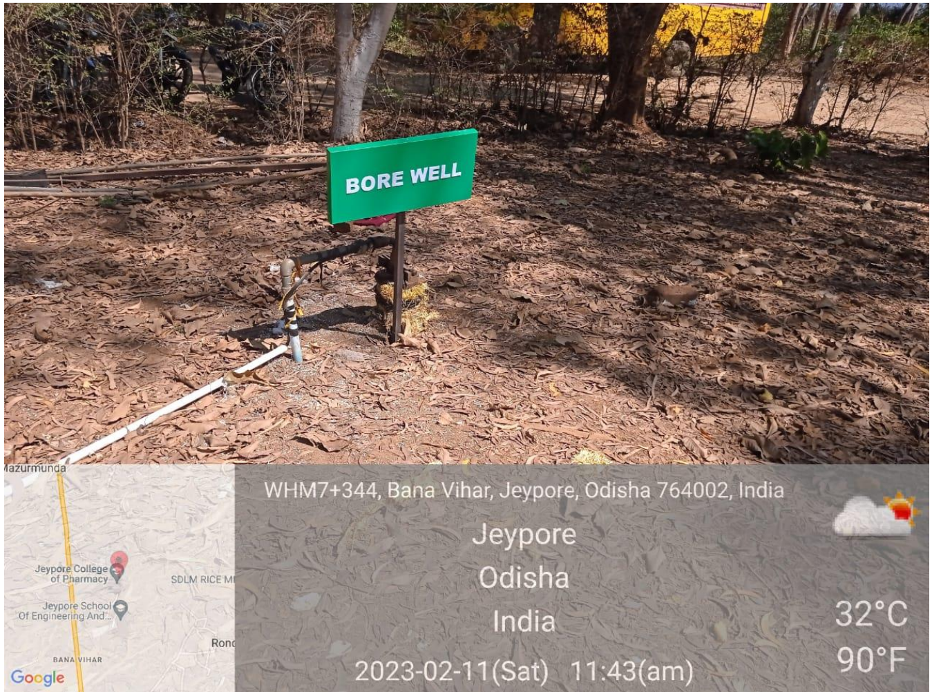
Fig-5 Bore well at JCP.
