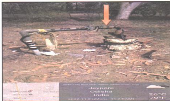
Fig:- 2.3 Requirement of water meter on bore well
